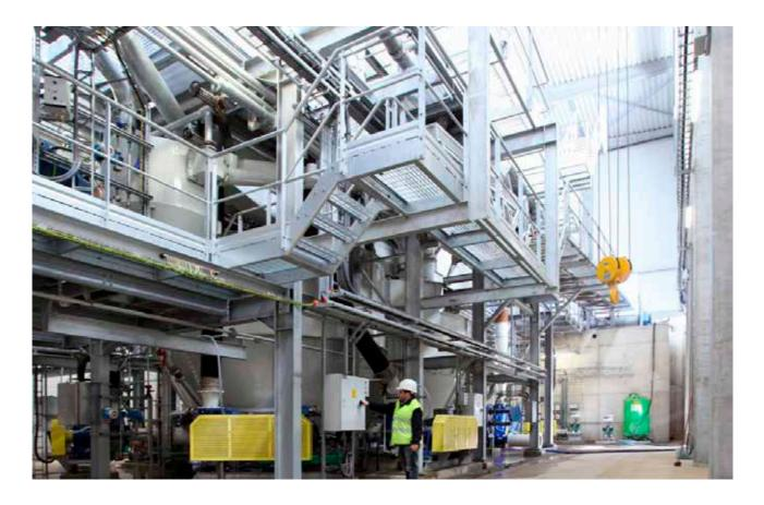
**PROJECT DESCRIPTION** Electrical installation of silt dewatering, board manufacturing and mounting, supply of EEx and non-EEx lighting boards and lighting installation, tracing, data wiring, tubing and cable runs, EEx and non-EEx instrumentation, support and commissioning.
